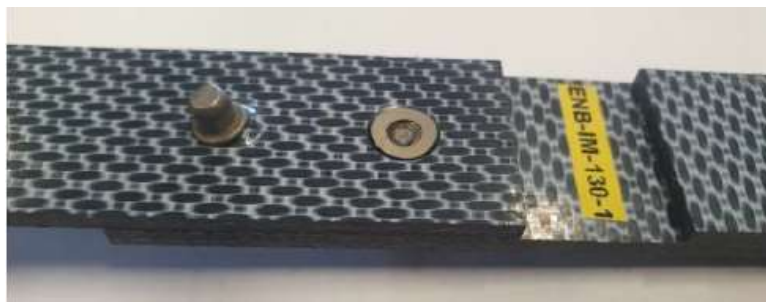
Figure 10 Example Failure Mode: Combination of Fastener Head Failure and Tilting/Laminate Bearing
