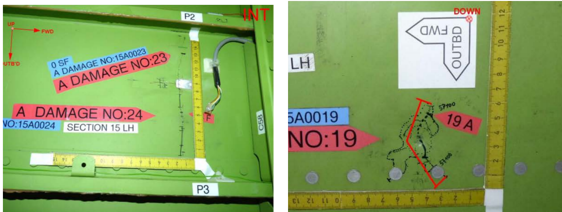
Figure 4: Fatigue cracking from deep fuselage dent.
